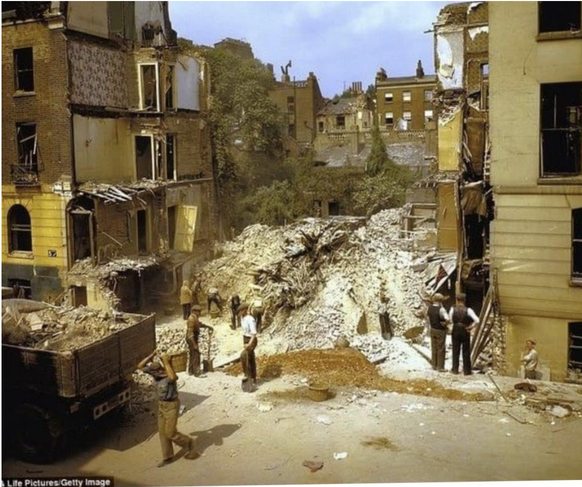
Workers removing rubble from building decimated after a heavy German air raid
